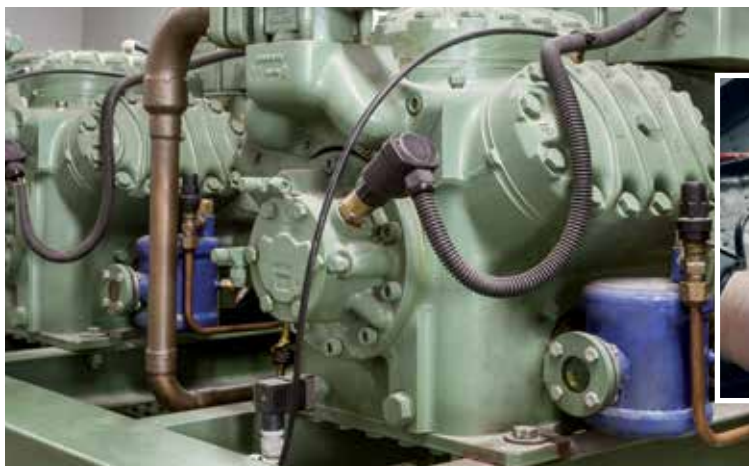
Presetting or adjustment of the pressure switch of a compressor
